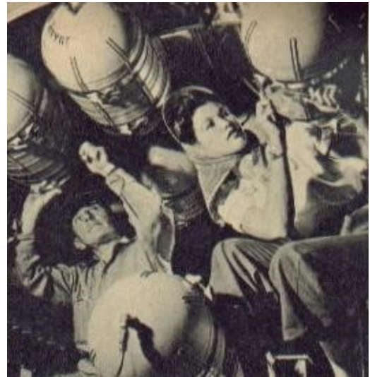
An altitude must is oxygen. Here workers of the Tucson Division complete installation of the main oxygen tanks. They feed various personnel spots.
